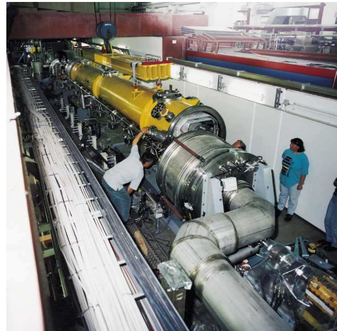
Superconducting accelerating module
